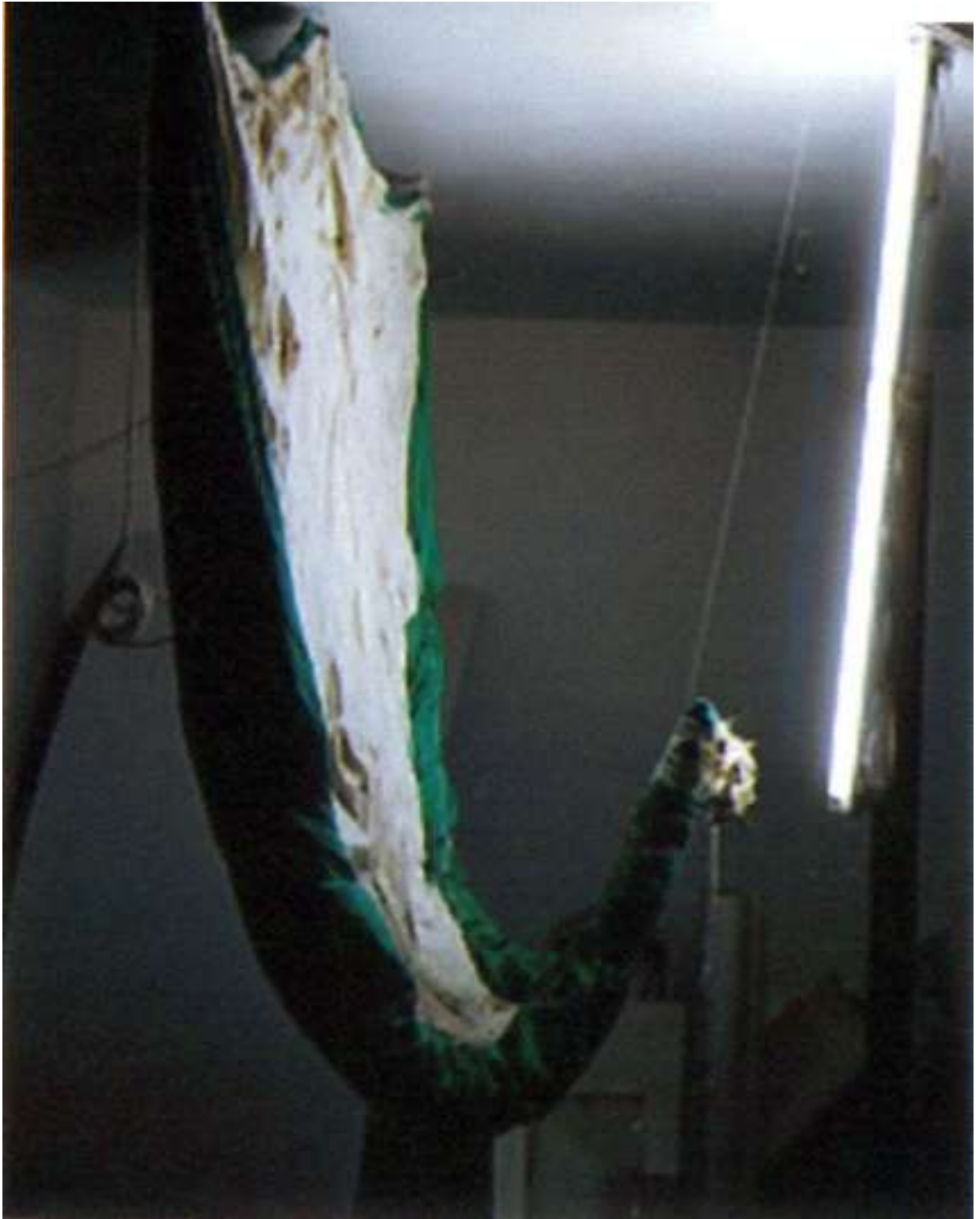
Installation detail-lights on
